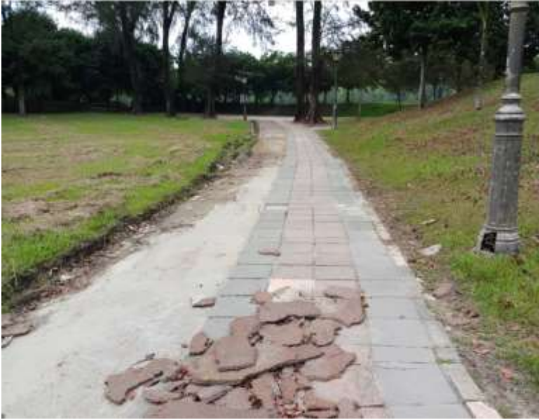
Broken tile everywhere at existing walkway/ jogging track.
